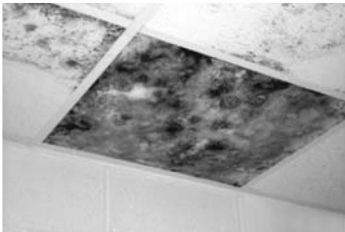
Moldy ceiling tile, thanks to a poorly insulated pipe.
