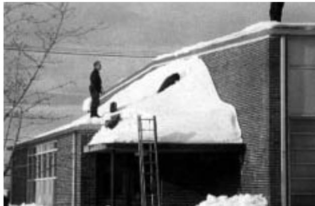
The peak snow load of this drift was 130 psf. The ground snow load at the time was 20 psf, and the snow load on the upper roof was 15 psf.
