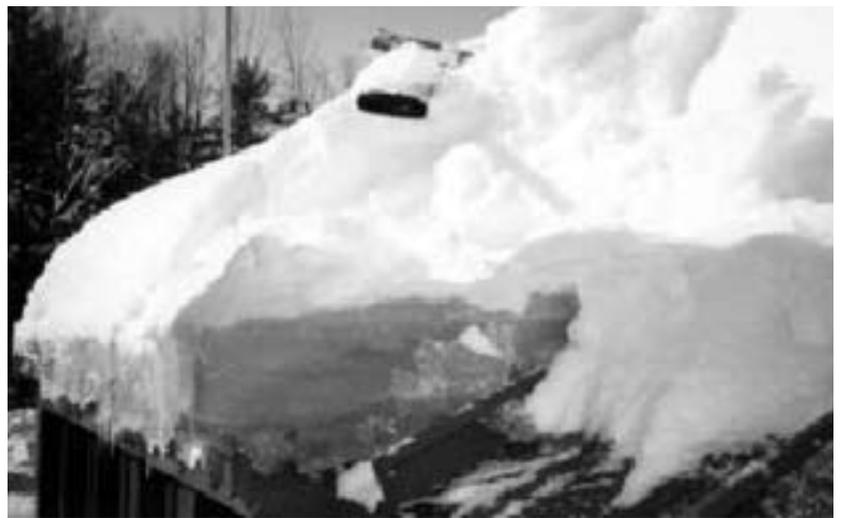
This large ice dam caused this metal roof to leak at its eaves.
